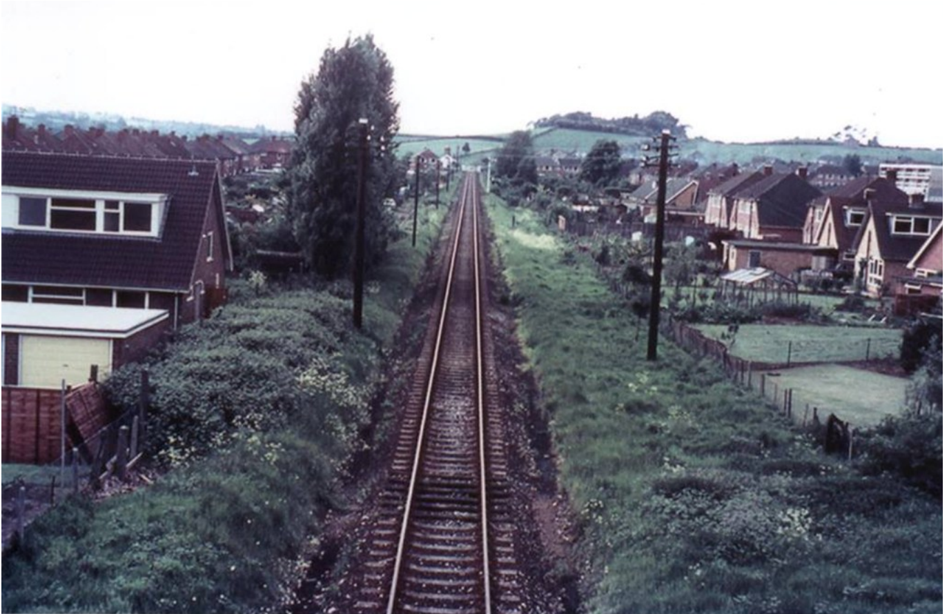
Looking north towards the site of the old Burlish Halt. In the distance are the Burlish Crossing gates
