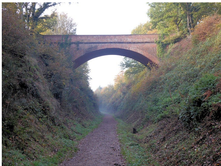
View from the railway cutting up to Wilden Top Road
