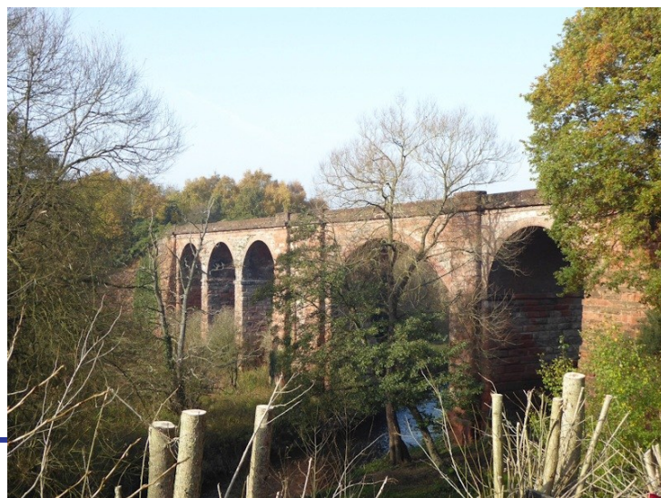
View of the viaduct over the River Stour and Stour valley
