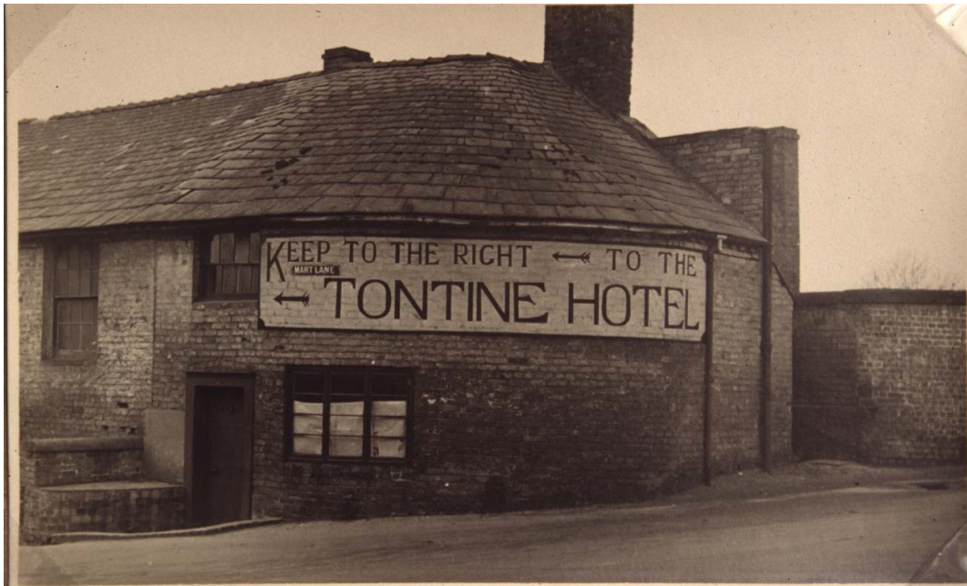
Curved end warehouse at end of Mart Lane
